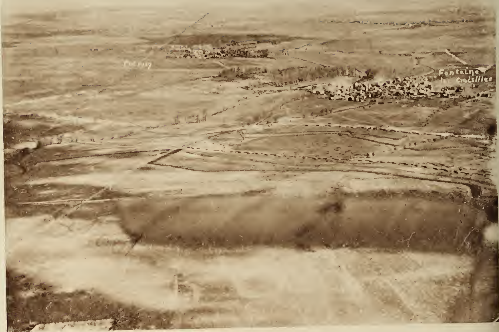
AEROPLANE PHOTOGRAPH SHOWING THE HINDENBURG LINE WEST OF FONTAINE-LES- CROISILLES.
